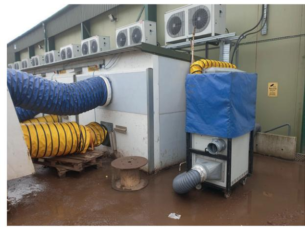
air then cycled back into the plant. Thanks to the skill of Polygon's technicians, a TCS1350 dehumidifier was incorporated into the plenum chamber set-up, enabling moisture to be removed from the sprouts while keeping temperatures at the low level required.
