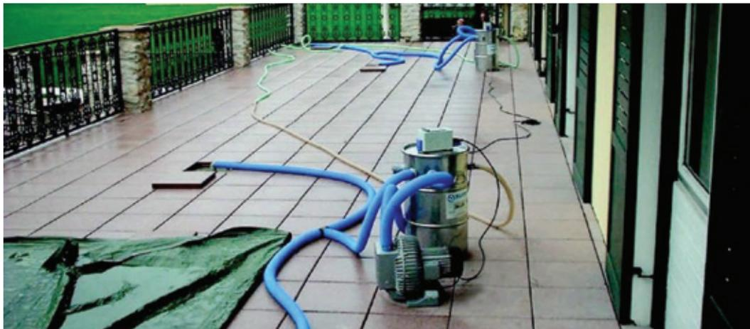
It is essential that dry air is allowed to flow through the insulation or the structure will not dry fully. This method is only suitable if the structure is free from dust and bad odour or the surrounding area will be affected. Turbines can be used to suck dry air through the structure to remove bad odour; with the wet air being released out of an open window or through a similar escape route. A dehumidifier is then used to dry the air in the room itself.
