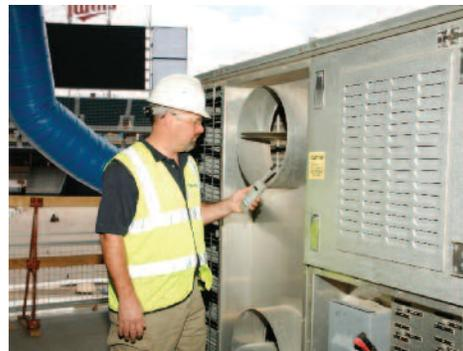
**To prevent warping and bending, HCU-6000 dehumidifiers were used to maintain the manufacturer’s specified conditions for the high-end millwork and construction materials.**
