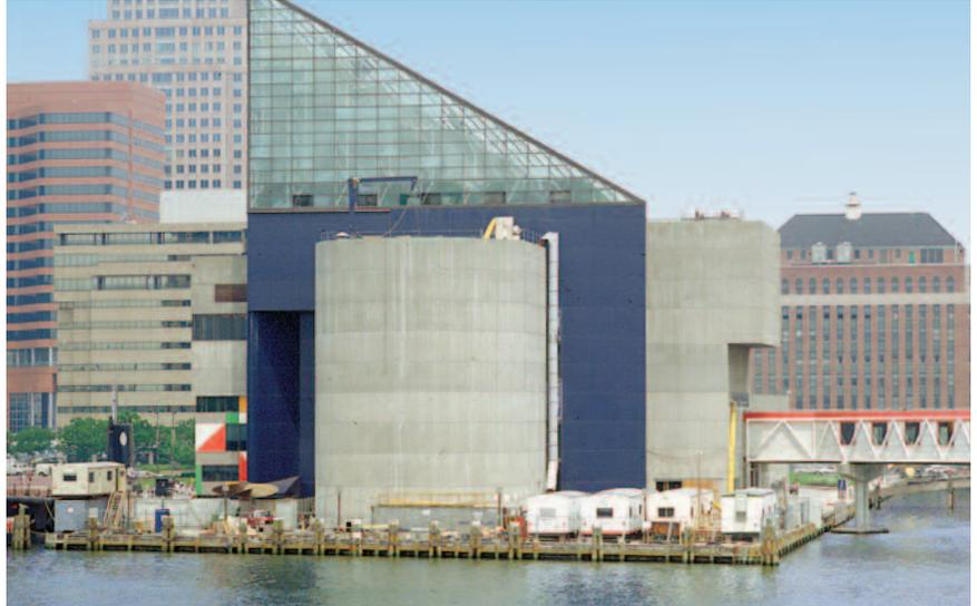
Handling a difficult site problem — normally, large dehumidifiers would have been used to dry the 130,000 cu. ft. tank at Baltimore's National Aquarium, but limited on-site space required a more flexible solution. Polygon's versatile fleet provided combinations of lighter and smaller dehumidifiers which could be positioned in available locations.
