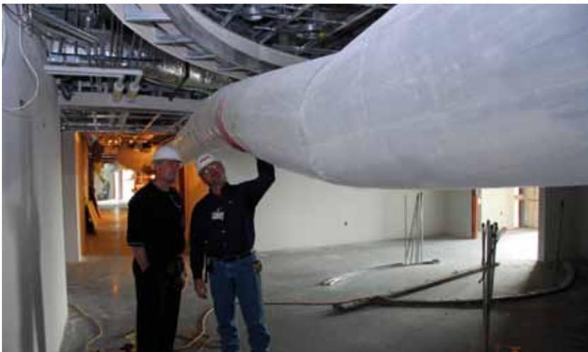
A flexible air distribution system was woven through stairwells and floors to reach all areas that required humidity control.
